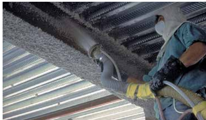
1.20 Application of a heat-insulating sprayed cementitious mortar layer. Any level of fire resistance can be achieved with this method.
