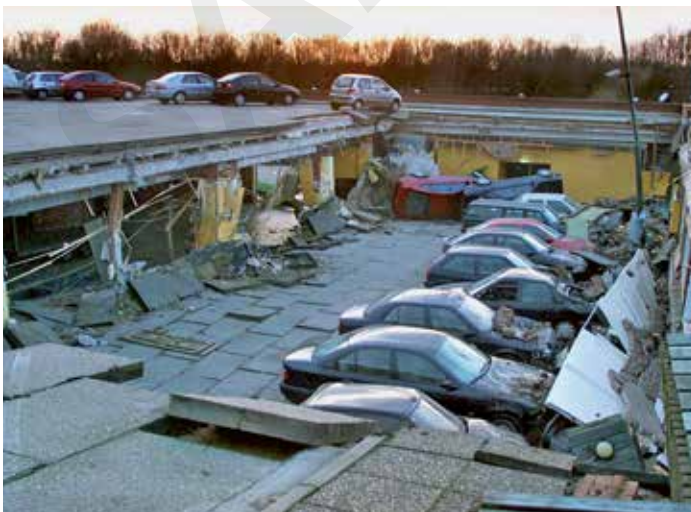
1.1 Collapsed parking deck at a hotel in Tiel (The Netherlands, 2002) due to, amongst other things, insufficient stability of the edge beam.
