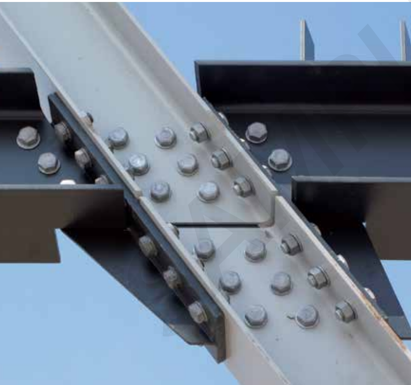
2.1 Example of a bolted connection.
