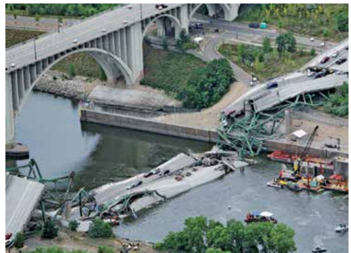
1.2 Collapsed Saint Anthony Falls Bridge in Minneapolis (USA, 2007) due to incorrectly designed joints (gusset plates) in the truss.
