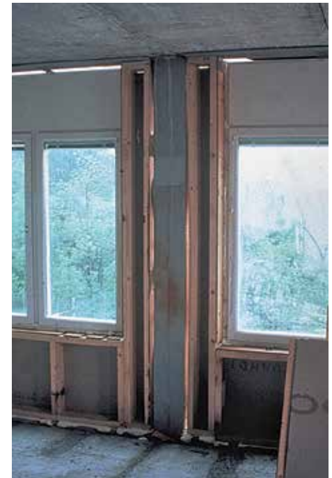
1.17 Integration of a steel column in a timber framed façade (covered with gypsum board on the inner side). Without additional measures, the fire resistance of the column is at least 30 minutes.
